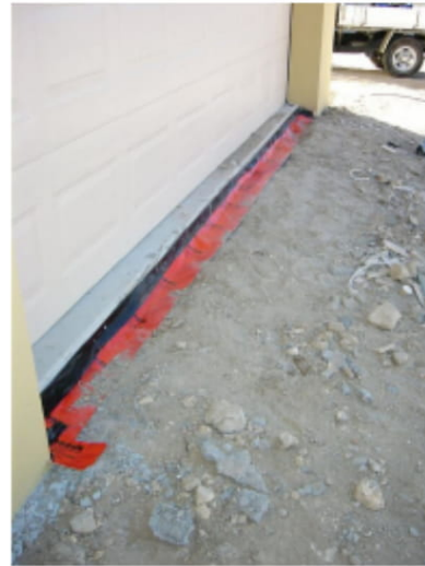
photo 2 garage entry detail
